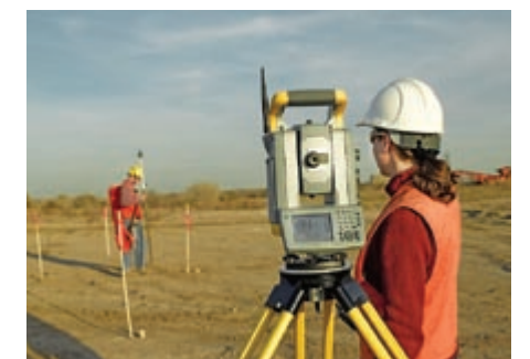
Stakeout and roading – automated stakeout of simple or complex projects.
